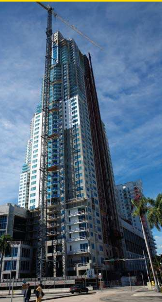
Everglades on the Bay in Miami, Florida, a luxury condominium project, used ProSpec Vertical Leveling Mortar to repair out-of-plumb walls, preparing them for a stucco finish coat.
