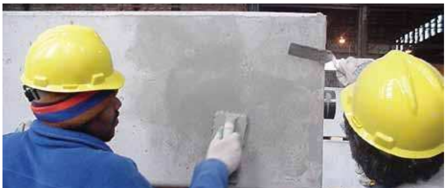
ProSpec RubCrete is used to repair bug holes and other surface defects in precast concrete.
