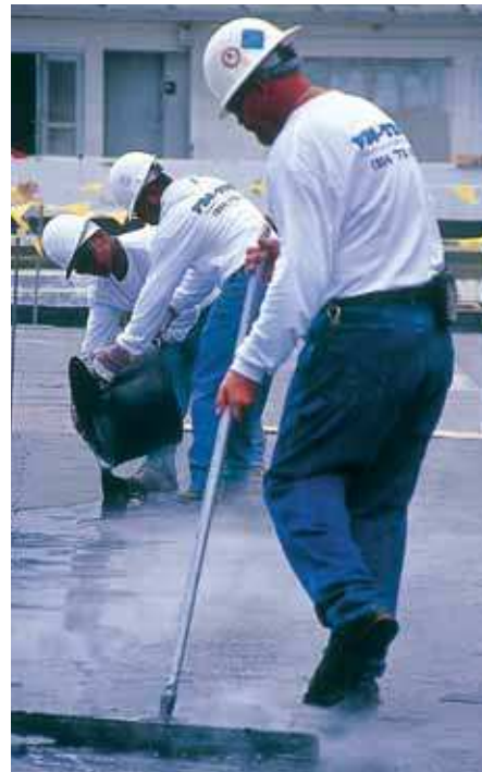
CCW-500R Waterproofing System is one of the essential components available for CCW Green Roofs.
