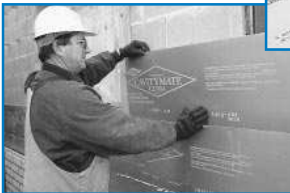
STYROFOAM CAVITYMATE Ultra brand insulation is installed directly between masonry wall ties, eliminating the need to cut or snap boards and ensuring a tight fit at the seams.
