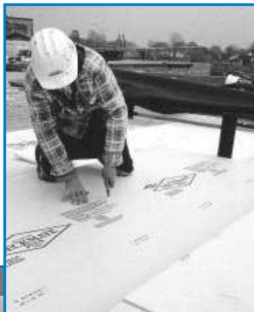
Two layers of 1½" STYROFOAM DECKMATE Plus brand insulation are applied directly to sloped and flat metal roof decks.
