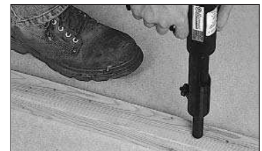
2" x 4" to concrete slab
