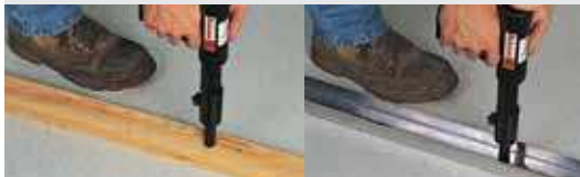
2" x 4" to concrete slab
