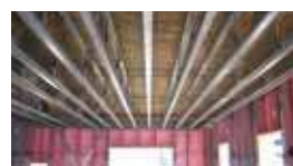
OSB and plywood to iSPAN joists
