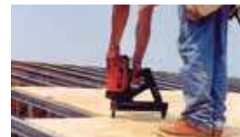
Plywood attachment—using TrakFast plywood to steel pin
