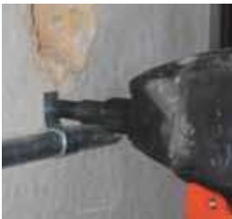
12HSMP034 clip assembly used to secure conduit
