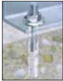
Fastening to Concrete with Threaded Rod
