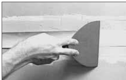
1. Fill Joint And Bed Tape Simultaneously
