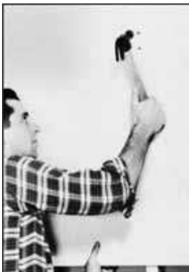
DOUBLE NAILING Minimizes nail-pop.
