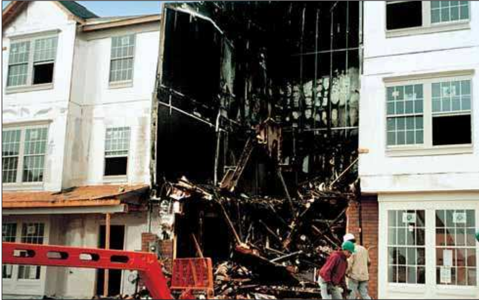
The fire-protection of gypsum-based Area Separation Walls is demonstrated in dramatic fashion by the results of this actual townhouse fire in which the two-hour fire-rated assembly performed as expected in protecting adjacent properties. Break-away feature allowed collapse of fire-side structural framing without pulling down the entire wall.
