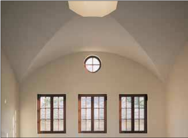
Veneer plaster expands architectural design limits as with this curved vaulted ceiling.
