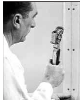
Joints are reinforced with Kal-Mesh fiberglass webbing. Steel corner and casing beads protect corners.
