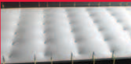
RhinoBond spreads wind load across the roof
