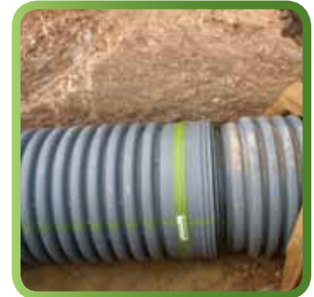
Bell/Spigot Joint Connection
