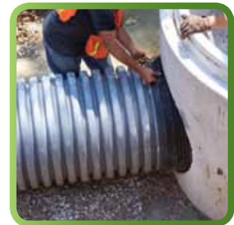
Manhole Boot Connection with Corrugated Pipe Adapter
