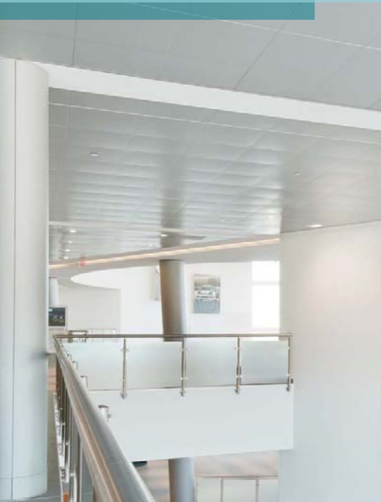
MetalWorks Torsion Spring 2' x 2' with M15 perforation in Silverlume on Prelude® Suspension System
