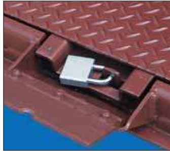
Recessed padlock hasp covered by a flush hinged lid
