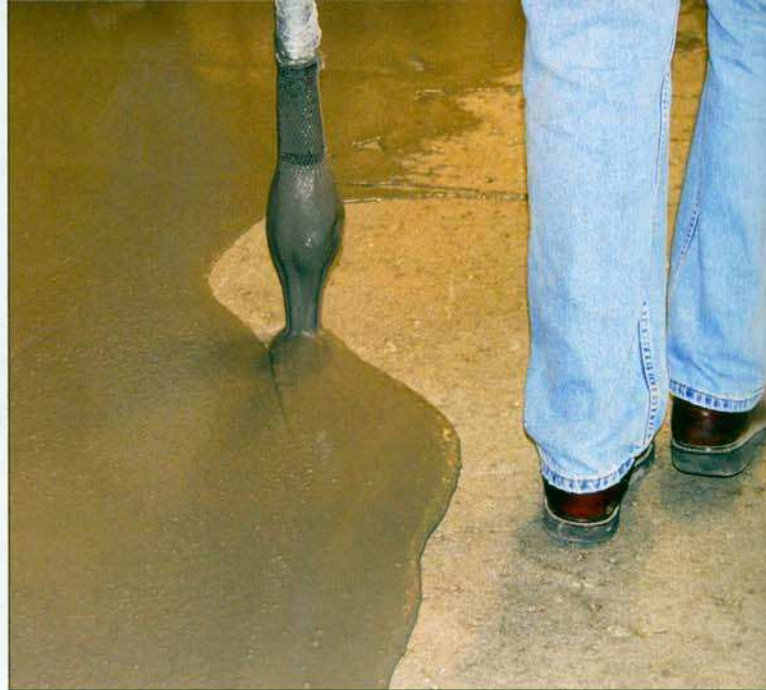
At left, a continuous mixing rotostator pump, utilizing a dustless vacuum system, is used to prepare the floor. The photo on the right illustrates how the 'sock' at the end of the hose on this rotostator pump catches unwanted material such as small lumps and pieces of bag.
