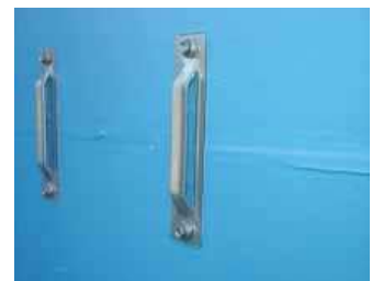
Installed using screws with neoprene washers
