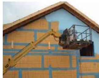
Barritech VP sprayed over joint details
