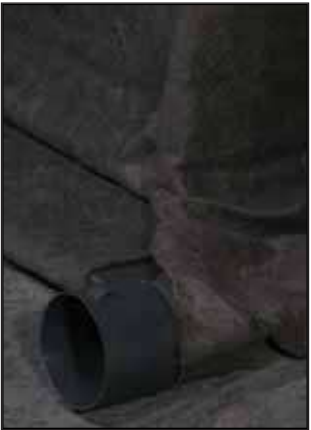
(B) 6" Endout Connector covered with fabric
