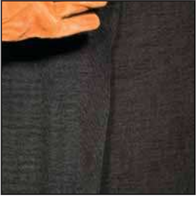
(B) Mate fabric flaps together and fold over adjacent panel. Adhere fabric with approved CCW adhesive.
