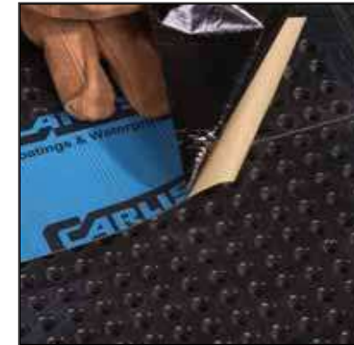
CCW MiraDRAIN joined top-to-bottom with 4" CCW-705
