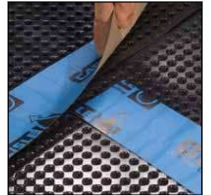
CCW MiraDRAIN joined in a "T" intersection with 4" CCW-705
