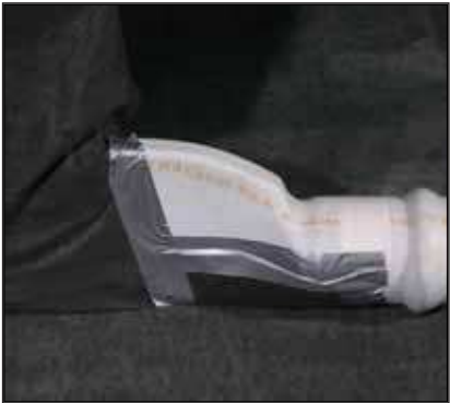
(B) CCW QuickDRAIN Connector attached to end of CCW QuickDRAIN & covered with extra filter fabric on cut edge and adhered with tape.
