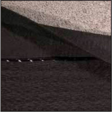
(B) The top or terminal edge of CCW MiraDRAIN should be sealed by applying a piece of filter fabric sufficient to prevent soil or other foreign construction materials from intruding into or behind CCW MiraDRAIN panels, an alternative would be to cut the core from the fabric by a depth of 3 dimples to provide excess fabric for wrapping behind the core.
