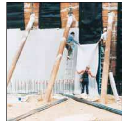
Soldier Pile Support with CCW MiraDRAIN and CCW MiraCLAY
