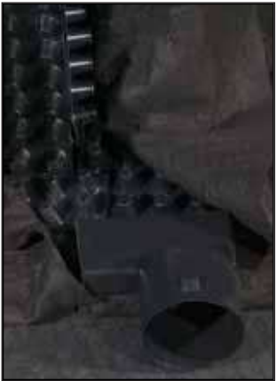
(A) 6" Endout Connector attached to CCW QuickDRAIN
