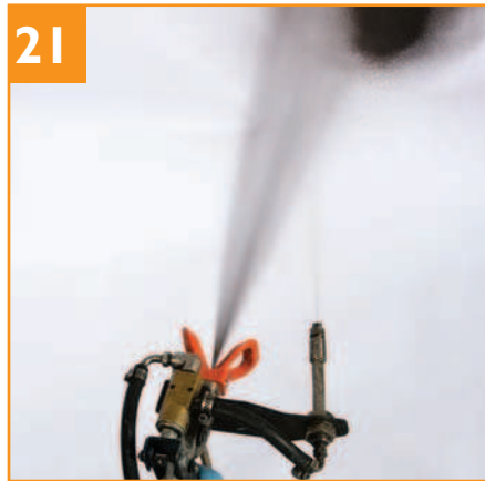
Spray Technique Operator shall spray with the nozzles positioned 20 to 24 inches from the surface. Spray lower area first, working upward. Keep spray direction square with wall surface. When sprayed properly, Barriseal-S/Barricoat-S should set up immediately, with fairly smooth surface texture and no running or blistering.
