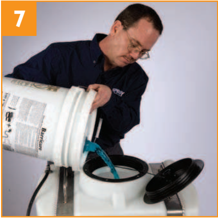
Pour full 5-gallon pail of Barricure into 25-gallon tank on Co-Spray Assembly.
