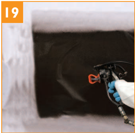
Good Even spray pattern. Pressure and nozzle size provide an even coating of spray without "fingering" or "ralley striping."
