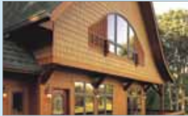
Fiber Cement Siding
