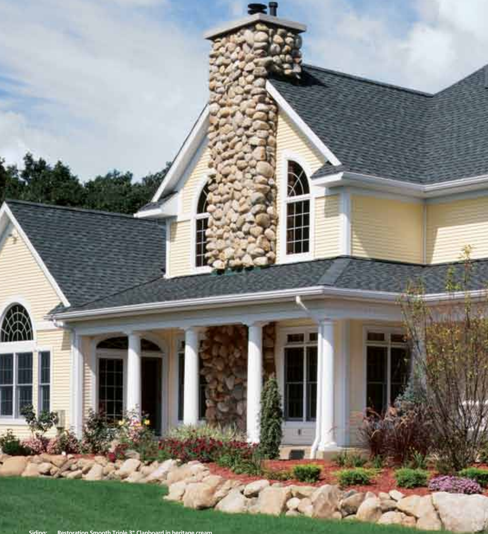
Siding: Restoration Smooth Triple 3" Clapboard in heritage cream. Trim: Vinyl Carpentry® & Restoration Millwork®.
