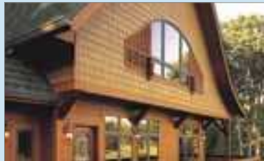
Fiber Cement Siding
