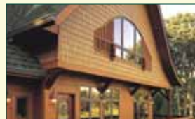
Fiber Cement Siding
