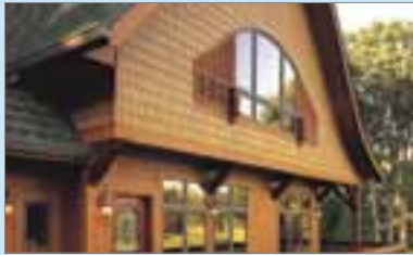
Fiber Cement Siding
