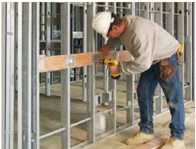
Secure each plate to the stud flange using two small pan or wafer head screws.
