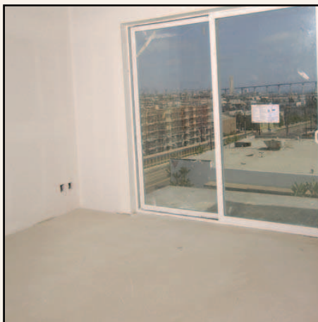
5 In as little as two hours after the underlayment has been poured, the floor is hard enough to accommodate foot traffic, so light subtrades may continue working. Total drying time varies depending on the type of finished floor goods to be installed, but is generally completed within 10 to 14 days.
