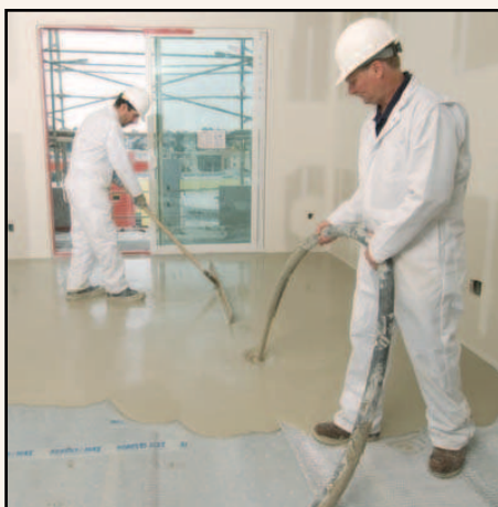
4 Sound mat is topped with approved Maxxon Underlayment, at a depth specific to the mat chosen for the application.* Installers use a "screed" to finish the underlayment surface. (If mat is installed only in hard surface areas, the underlayment is poured directly over the subfloor in areas to be covered in carpet and pad.)
