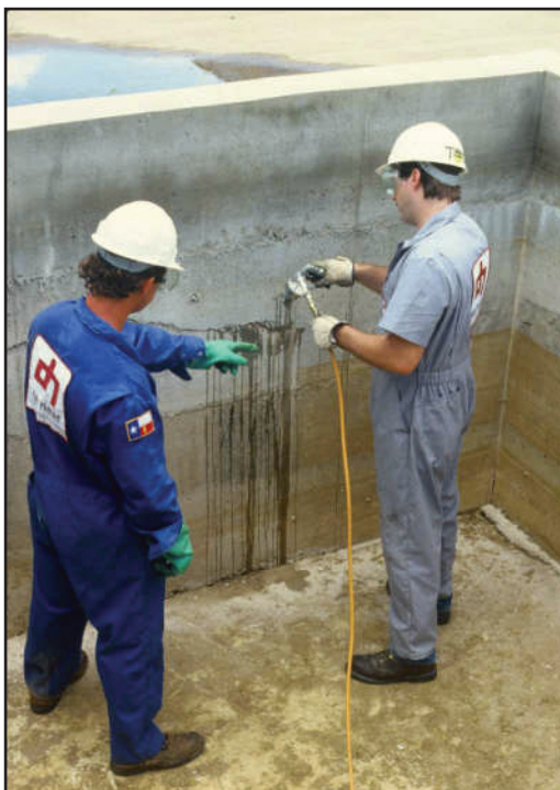
(STEP 6. FLUSH CRACK)
