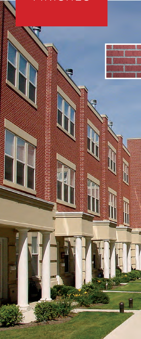
Brown Street Station Condos, Chicago, IL
