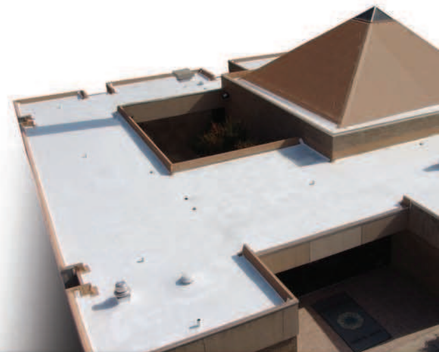
Duro-Last Roofing System Prefabricated Membrane Sheets Lineal Feet of Field Seams - 1,278
