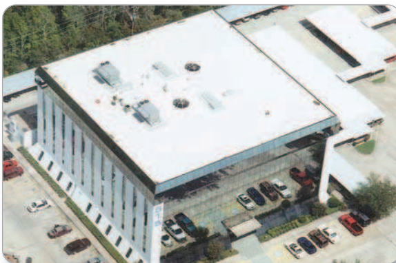
Complete roofing system
