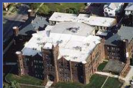
Castle On The Hill in Sioux City, Iowa Installed by Nohava Construction, Co.
