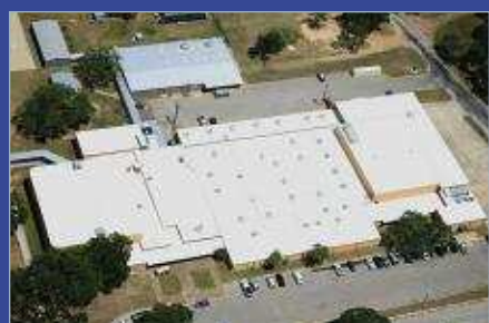
Columbus High School in Columbus, Texas Installed by Jaco Construction
