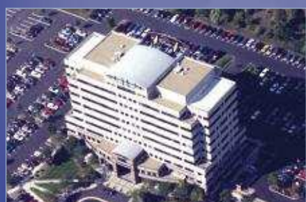
Gates-McDonald Office Building in Hilliard, Ohio Installed by Chemcote Roofing, Co.
