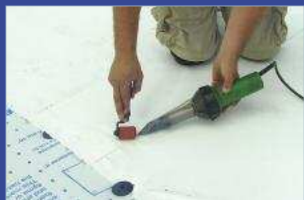
Roof Installation in Saginaw, Michigan.
