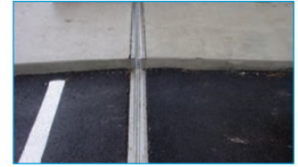
DSM-FP is a versatile expansion joint for split-slab construction as well as split slab-to-solid slab applications. Fabricated transitions from deck to wall, at curbs, sidewalks, parapets, tees, and crosses are available with the DSM-FP.
