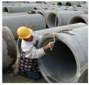
production and installation process, there is the possibility of honeycombs or chipped surface areas that need to be repaired with either a coating or patching compound. In addition, refurbishing of existing precast structures is commonly required to repair scaled or spalled surfaces that are incurred from everyday wear and tear.
