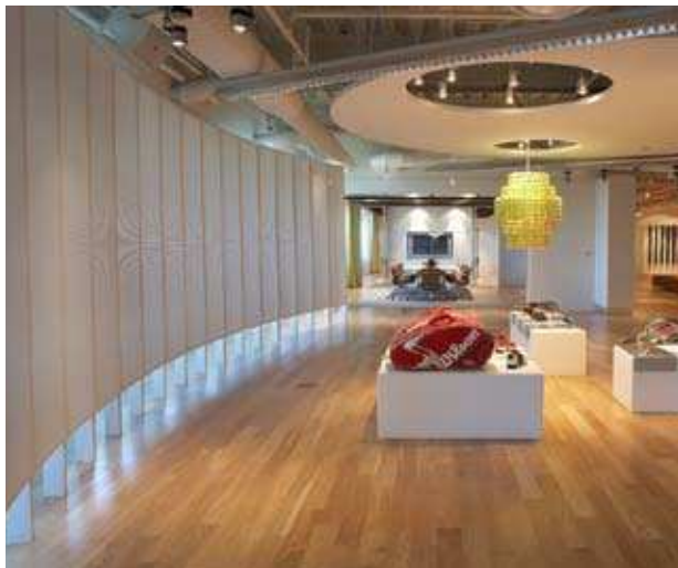
Fry Reglet Acoustical Wall Panels secured to aluminum posts are used as a projection screen at Wilson Sporting Goods facility.
