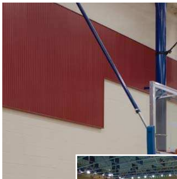
Fry Reglet Acoustical Wall Panels reduce echo and add to the aesthetics of gymnasiums.
