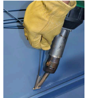
Step 4 - Permanently weld with secure rod
