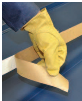
Step 3 - Remove tape/ affix to membrane
