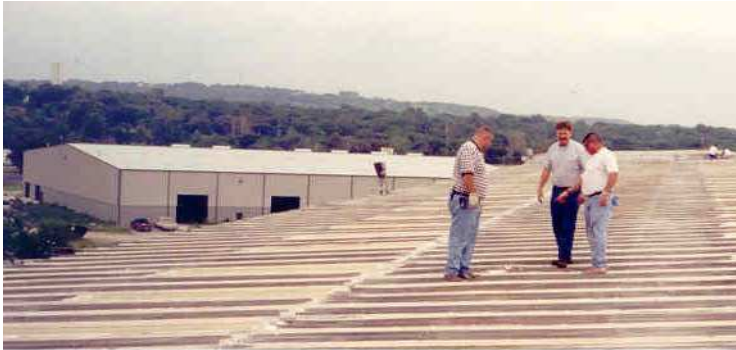
David Kummers, John Suskey, and Alan Lewis check over the prep work on the skylights and metal roof before the application of Inland Rubber Roof Coatings
