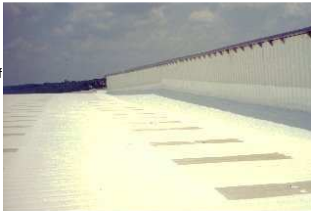
A total of 292 fiberglass skylights were protected with Inland's CR-2100 Skylight Coating
