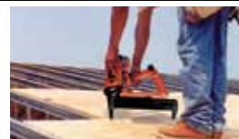
Plywood attachment—using TrakFast plywood to steel pin
