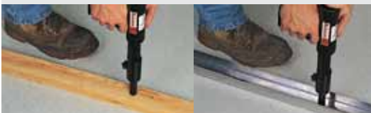
2" x 4" to concrete slab
