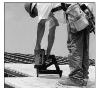
Plywood attachment—using TrakFast plywood to steel pin
