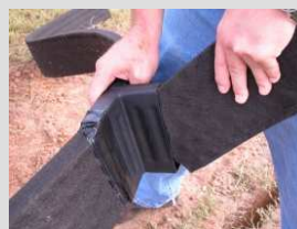
Inserting into fitting/tape
