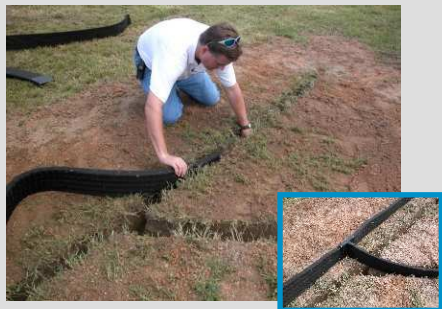
Installing J-DRain SWD-6 into shallow trenches
