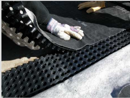
Figure 1. J-DRain GRS core has inter-locking dimples
