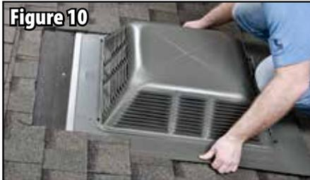
7. With the side marked UP aimed toward the ridge, carefully slide the unit into place allowing the motor wiring to hang down into the vent opening. Align the center marks on the flashing to the center marks made from the template, this will ensure that the throat of the unit is centered over the vent opening. See figure 10.
