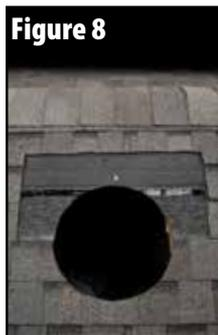
5. Trim and remove shingles inside the marked trim line. **DO NOT CUT FELT PAPER.** Carefully remove roofing nails from the surrounding area so the flashing of the unit will slide under shingles. See figures 7 and 8.
