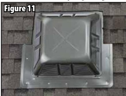
8. Fasten the base to roof decking with roofing nails, keeping heads of nails under shingles where possible. See figure 11.
