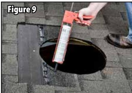
6. Apply roofing cement around the edge of the vent opening. See figure 9.
