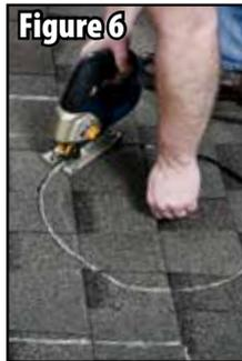
4. Drill a pilot hole inside the marked hole position. Insert the saw blade in the pilot hole, follow the hole pattern and cut out the 16" vent opening. See figures 5 and 6.
