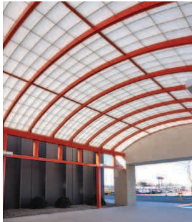
Fleet Farm - Owatonna, MN Widseth Smith Nolting
