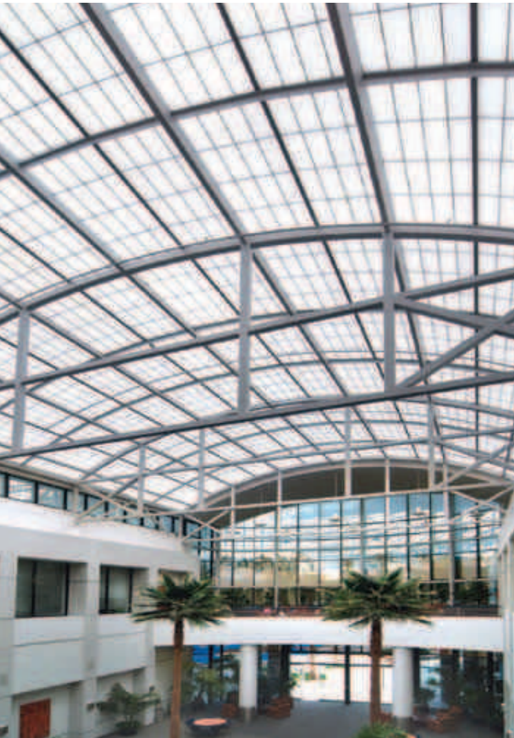
Gen-Probe PHASE II - San Diego, CA Smith Consulting Architects
