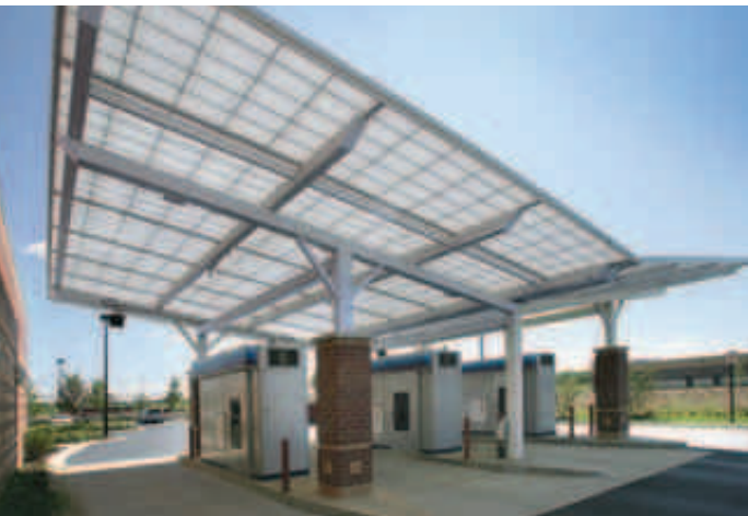
Citibank - Hoffman Estates - Hoffman Estates, IL Clune Construction Company
