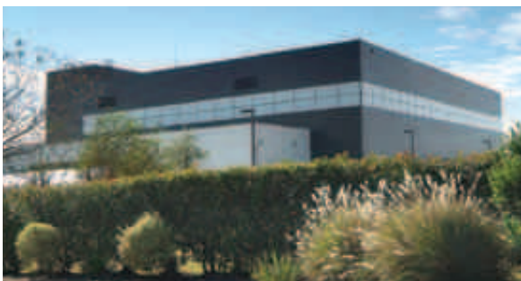
Aramco Hanger & Facilities - Houston, TX
