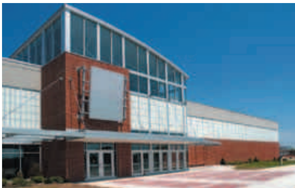
Cedarburg High School - Cedarburg, WI Plunkett Rayisch Architects
