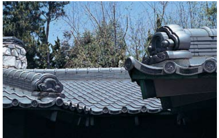
Re-Roof Project, Encino, California — Japanese Black C09
