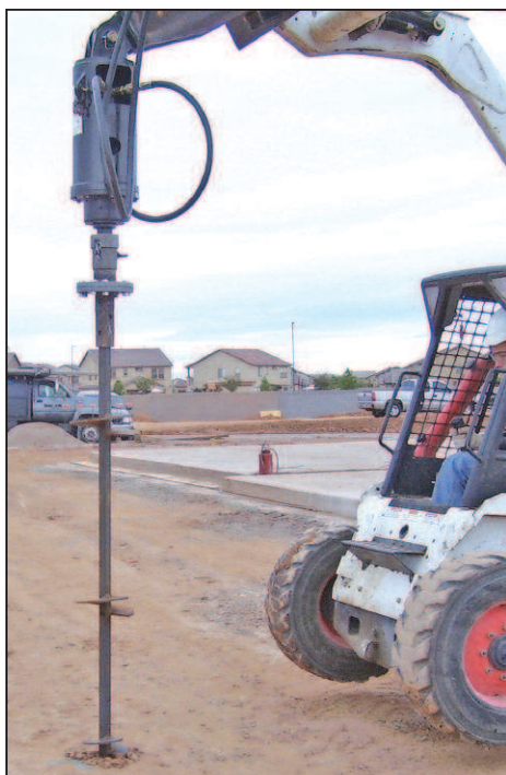
Typical MB Brace Badger Installation
