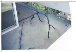
4. The largest cracks that appeared to be working and leaking directly through the topping slab and "T" slab were routed out with a crack chaser and filled with a pliable sealant.
