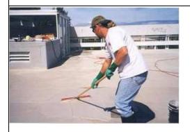
5. Next, the process of applying the first "scratch" coat of Miracote Protective Coating to smooth and fill surface voids.
