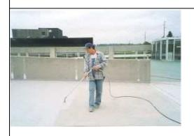
9. The final step in the system was the application of two coats of Miracote Colorbond Sealer. This can also be followed by an application of Miraseal.
