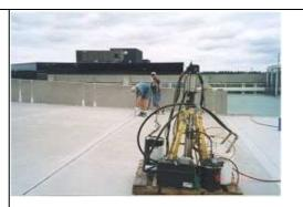
7. The membrane was then covered with three coats of Regular Miracote Protective Coating.
