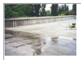
1. The first part of the project was pre-paring the surfaces. This included removing and storing for future reinstallation all of the pre-cast parking bumpers, then pressure washing the entire top deck.
