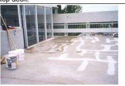
3. The low spots in the flat areas of the deck were then filled with Miracote Repair Mortar to eliminate ponding.
