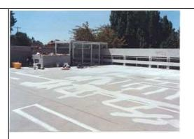
2. The next step required repairing all cracks larger than 1/16 inch with Miracote Protective Coating and imbedded fiberglass tape.
