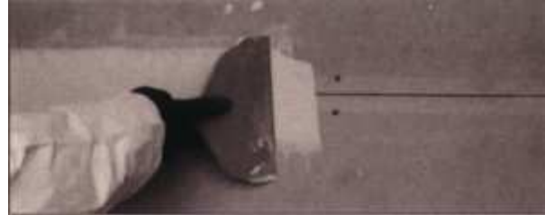
TAPE & MUD DRYWALL SURFACE SAND AS IF TO RECEIVE PAINT
