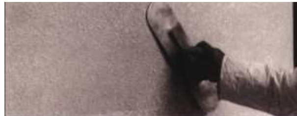
"KNOCK DOWN" WITH STAINLESS STEEL TROWEL
