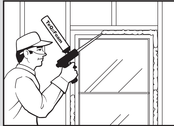
(Figure 11) TeQ::Foam™ application
