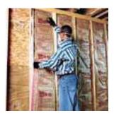
Note: Never leave faced insulation exposed. The facings on Kraft-and-foil-faced insulation will burn and must be installed in substantial contact with an approved ceiling, wall or construction material to help prevent the spread of fire in the wall, ceiling or floor cavities. Unfaced fiber glass is non-combustible.
