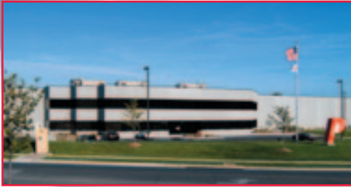
Headquarters and Plant in Omaha, Nebraska
