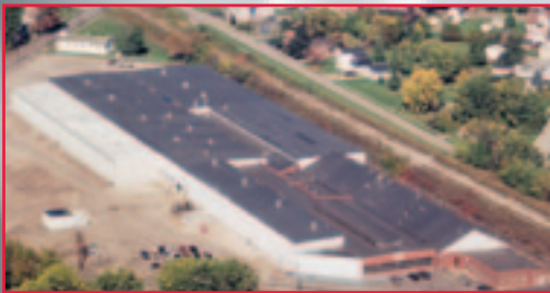
Office and Plant in Niles, Ohio
