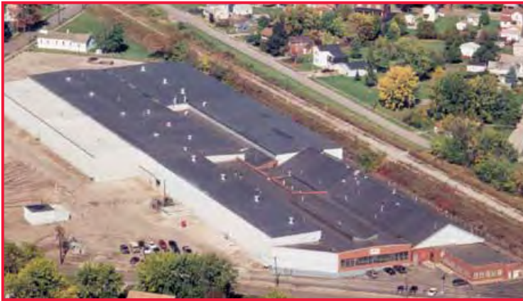
Office and Plant in Niles, Ohio
