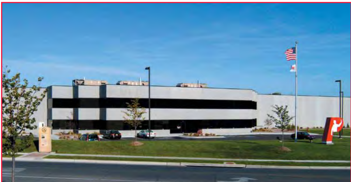
Headquarters and Plant in Omaha, Nebraska
