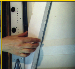
Insert the excess insulation behind the vertical rails
