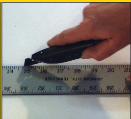
Cut each insulation sheet to length
