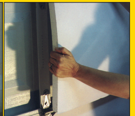
Insert the insulation sheet between the horizontal & vertical rails
