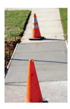
primarily because supporting soils have failed. Erosion, poor compaction, and decomposition of organic material all contribute to slab settlement.
