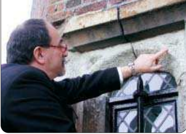
Assessing deterioration of Reigate stone at a project in the UK.
