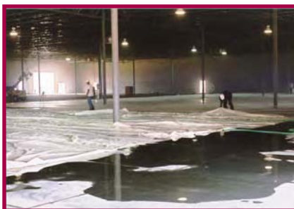
Re-wetting may be performed by the use of a soaker hose or equivalent.
