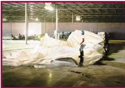
Wet the exposed concrete.
