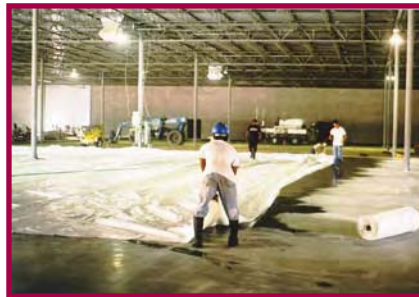
Apply Transguard® curing covers.
