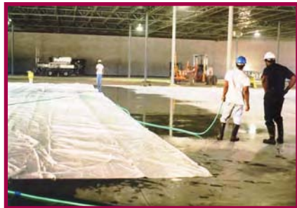
Check daily for proper moisture content.
