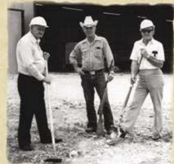
Owners Curtis Blackwell, Joe "Jody" Reeves and Preston Reeves breaking ground on a new building in 1979.
